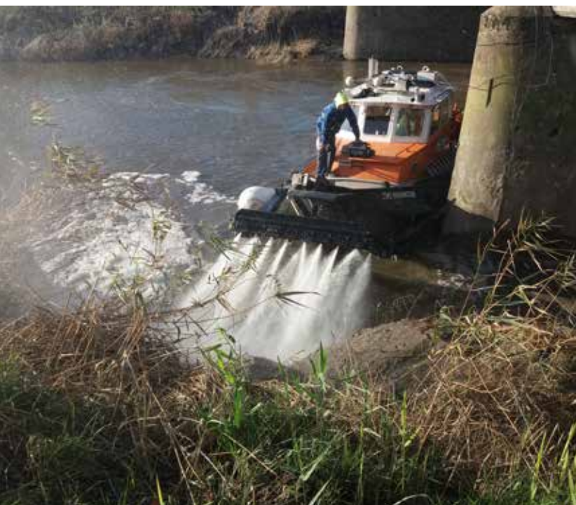
De-silting operations at Blake Bridge in Bridgwater
